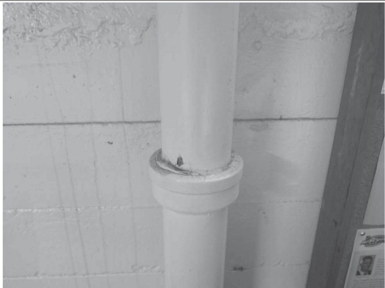
Picture No. 10: Suspect Asbestos in Gasketing on Pipe Bell and Spigot Packing
