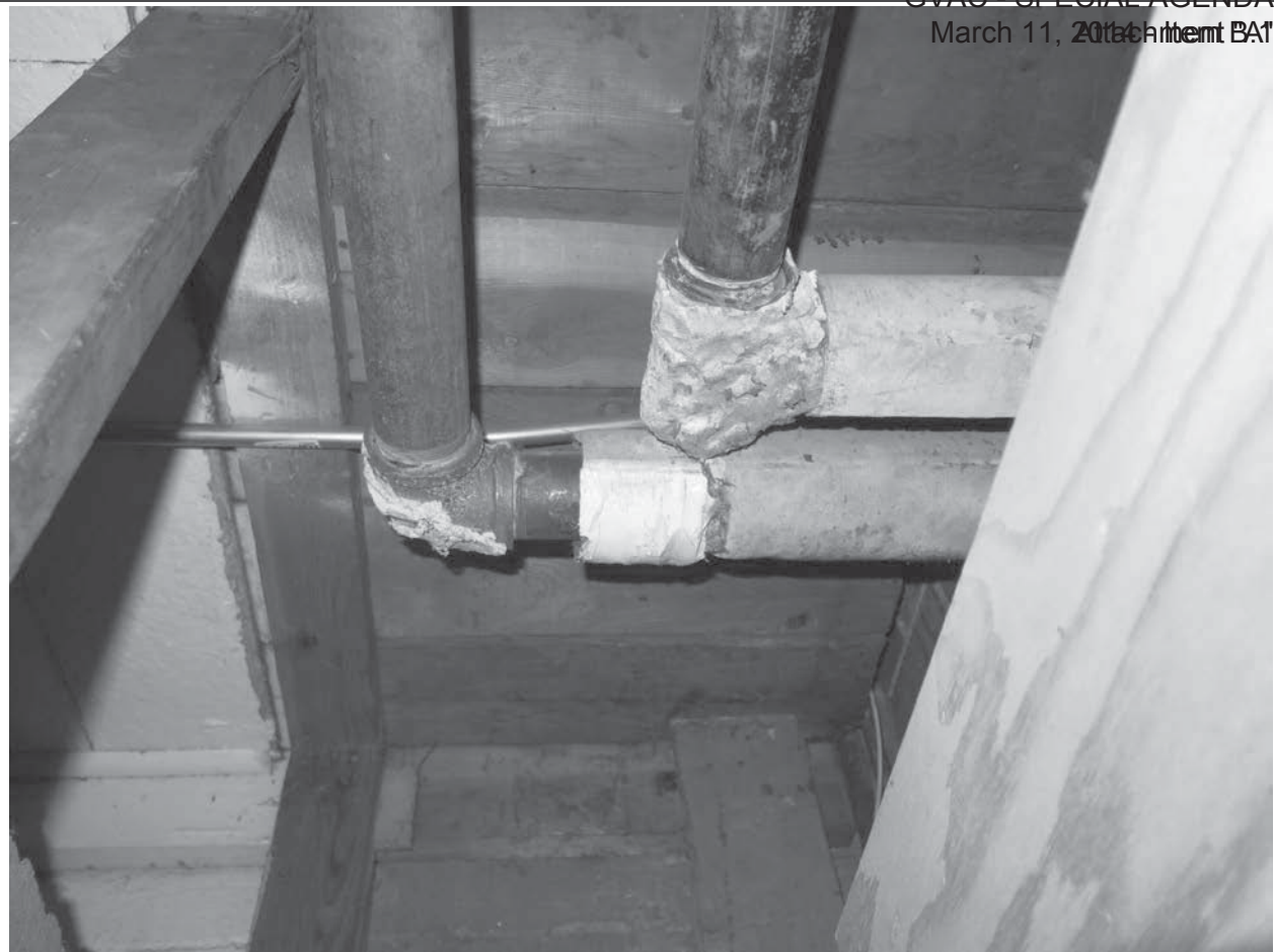
Picture No. 15: Poor Condition Asbestos Insulating Cement (typical)
