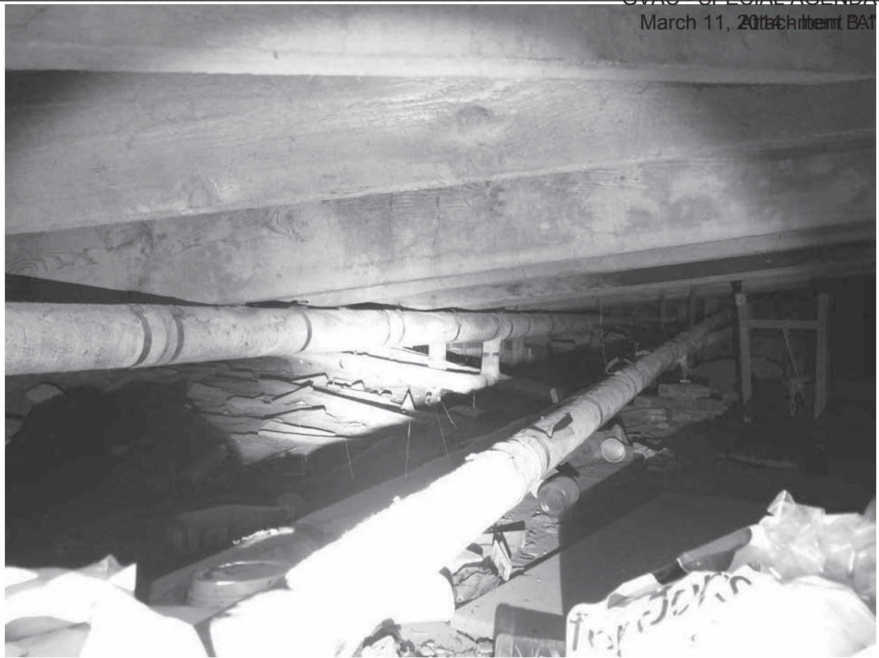
Picture No. 19: Asbestos Insulating Cement on Hot Water Heating Lines in North Crawlspace
