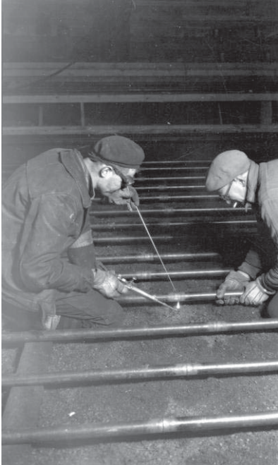
Above: Historical photo of the refrigeration piping being welded in situ Below and right: Refrigeration pipe during a recent repair
